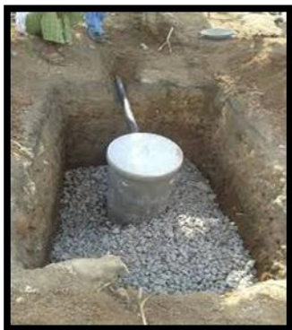
Construction of Soakage pits
